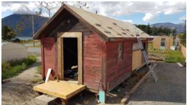
The Blacksmith Shop, with work in progress. Credit: Derek Crowe
